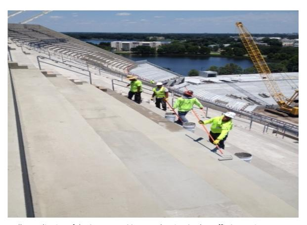
Roller application of the Strongcote SC-111 Pedestrian Grade Traffic System in two coats provide traction and protection of the concrete treads and risers of the upper bowl of the stadium  $\,$ .
