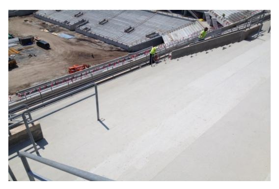
Above is a view of the completed section of the upper bowl where 240, 000 square feet of Strongcote SC-111 Pedestrian Guide Traffic Deck coating was applied during the renovation of this stadium.
